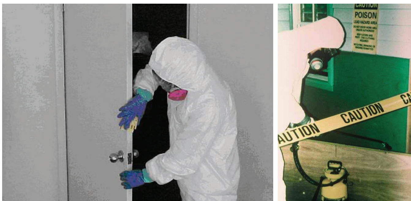
FIGURE 11.15 Stabilizing paint on doors: Wet planning (left) and wet sanding (right) deteriorated paint can create significant amounts of dust.
