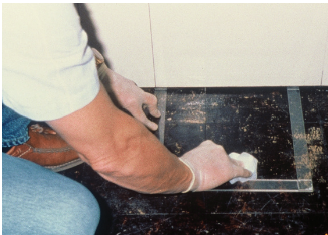
FIGURE 5.11c Making a first (horizontal) pass.
