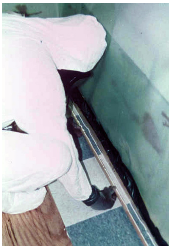
FIGURE 13.1 Encapsulating a floor with vinyl tiles
