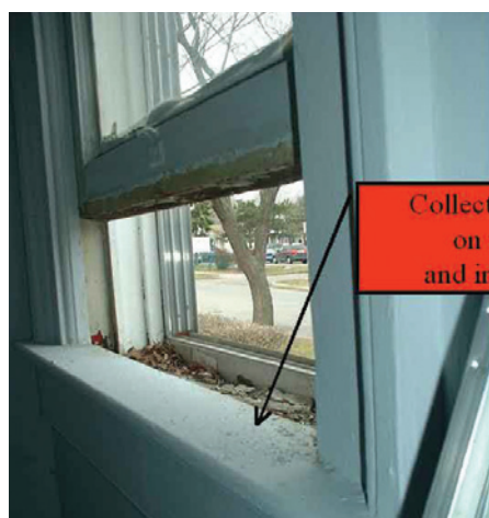
FIGURE 5.13 Window sill (at arrow); trough is behind sill, under sash and in front of storm window tracks.
