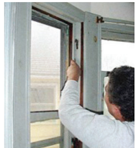
FIGURE 11.6 Remove parting Aboard.
