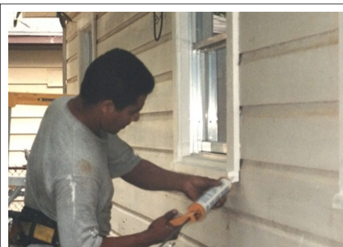
FIGURE 3.3 Worker caulking painted surfaces as part of ongoing lead-safe maintenance.
