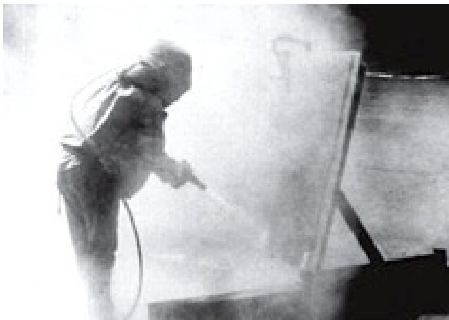
FIGURE 12.13 Prohibited work practices (traditional abrasive blasting (left) and grinding without HEPA exhaust).
