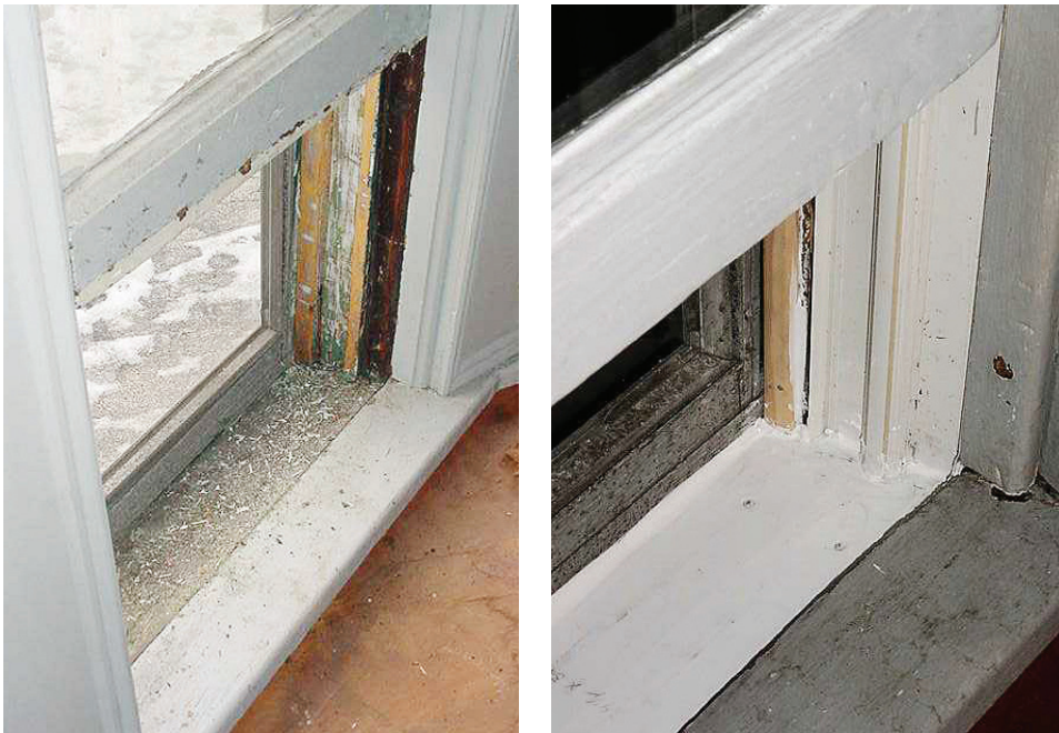
FIGURE 11.3 Window before and after friction treatment.
