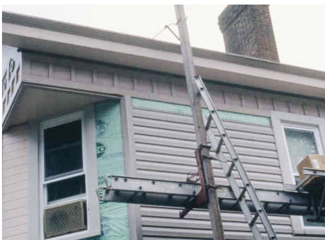
FIGURE 12.6 Installation of replacement siding.
