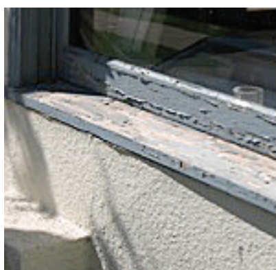
FIGURE 5.4a Peeling paint
