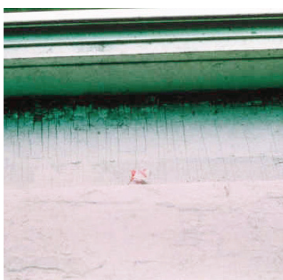
FIGURE 5.4b Alligatoring paint
