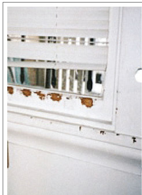
FIGURE 5.8 Chewable surface: teeth marks on window sill.
