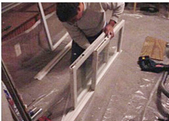
Figure 11.13 Fit sashes into jamb liners.
