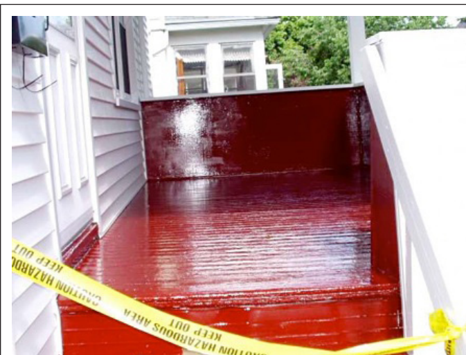
FIGURE 8.16 Example of barrier tape used as an occupant protection measure.
