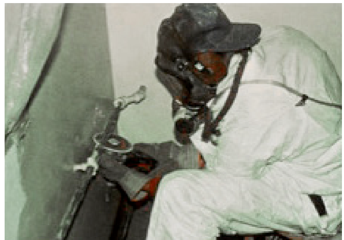
FIGURE 12.13 Prohibited work practices (traditional abrasive blasting (left) and grinding without HEPA exhaust).
