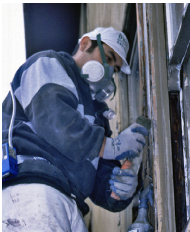
FIGURE 12.16 Wet scraping (left)
