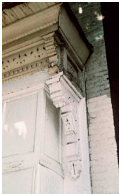
FIGURE 13.3 Encapsulated historic components.
