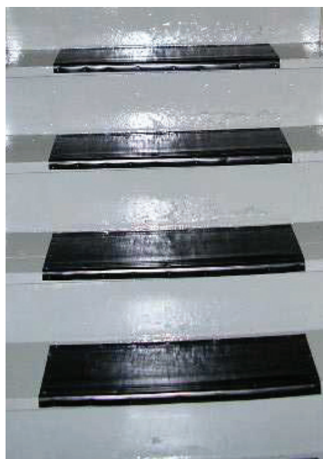
FIGURE 5.6b Friction hazard on stairs post-treatment.
