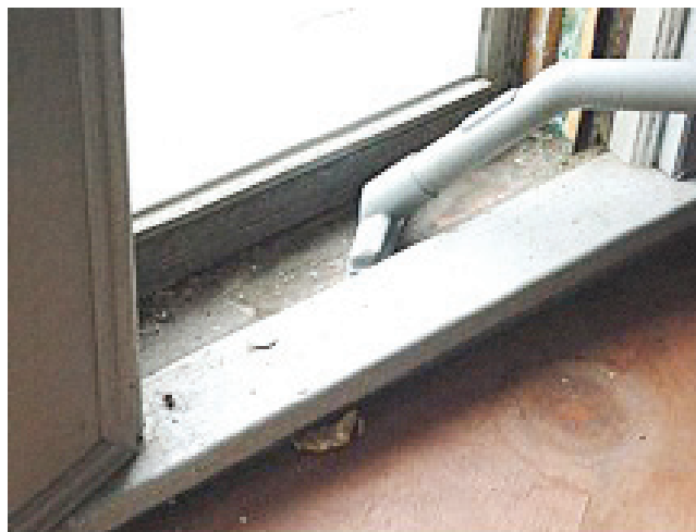
FIGURE 11.5 Prepare the worksite and pre-clean the window.
