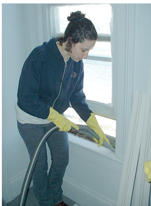
FIGURE 8.17 Pre-cleaning window with HEPA vacuum.
