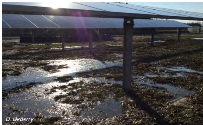
Figure 2-2: Example of surface water ponding on poorly-drained and compacted soil at a solar facility during construction.
