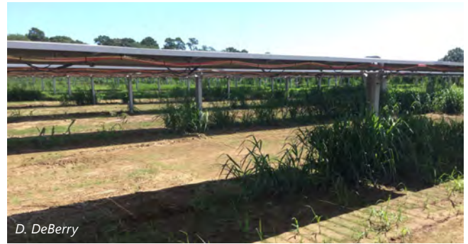
Figure 2-5: Example of soil compacted by heavy equipment, with minimal vegetation growth due to the surface soil compaction.
